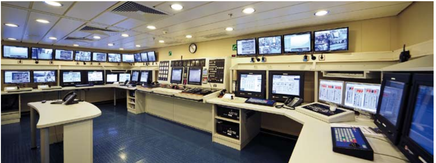
Engine Control Room of the "Celebrity Solstice"
