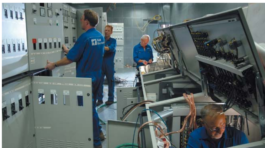
Installation of an engine control room
